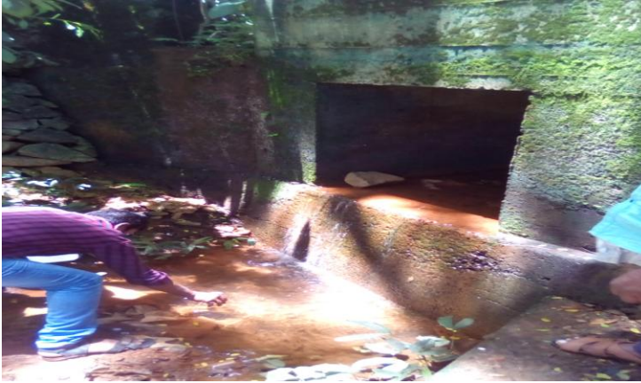
Fig 16. Odangad fish market side drain
